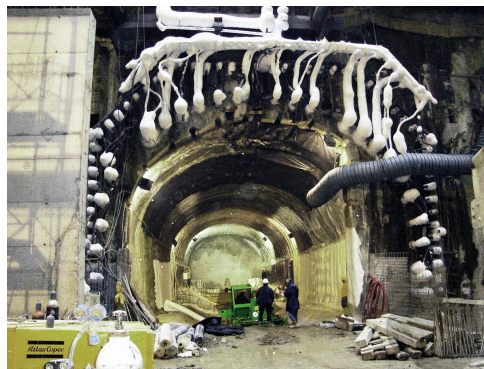
Figure: AGF in Naples underground line 1 – Garibaldi station.
